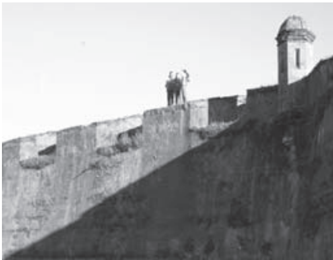
The Fortress of Corral in Valdivia, Valdivia’s system of fortresses, also known as the Key of the south sea, it is a set of fortifications placed in Corral, Niebla and Isla Mancera, At Valdivia’s bay. It was one of the biggest fortifications built by the Spaniards in America.
